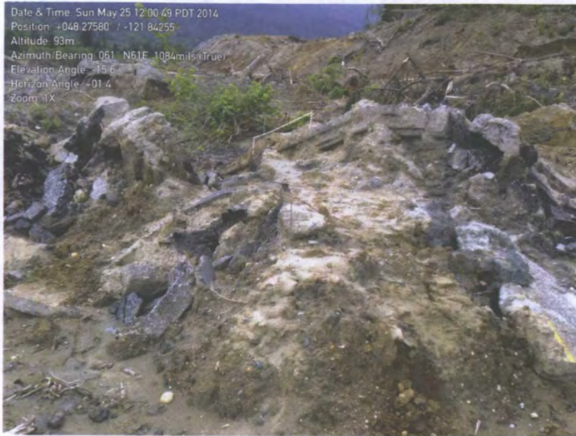
Figure 5.2.32 Asphalt with intact base course from SR 530 road bed plucked and transported by the debris flow. Note piece of asphalt in lower right with yellow paint stripe. Camera position: 48.27580°N, 121.84255°W, view to the northeast.
