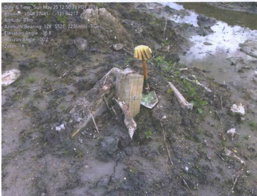
Figure 5.2.34. Section of guard rail (top) and timber support (bottom) transported from SR 530 by initial debris flow. Camera positions: 48.27478°N, 121.84196°W, view toward southeast (top); 48.27481°N, 121.84217°W, view toward southeast (bottom).
