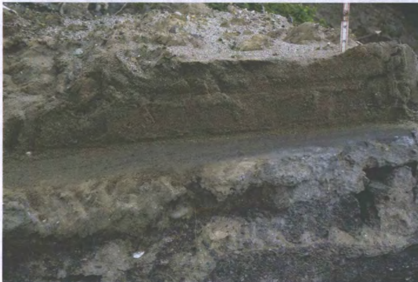
Figure 5.2.35. (upper) Example of one of several Highway 530 pavement sections that were uplifted and transported by the landslide. The pavement section (which is inclined down to the left) shows an intact segment of what is believed to be the first material to have crossed the highway prior to its subsequent uplifting and transport. The scale shown is in feet (location: -121.842560, 48.275860). (lower) Close view of the deposit above the pavement section. The photograph shows a course-grained tan sand over a thin (several mm) film of grey silt and clay over the asphalt. The pavement is underlain by a gravelly pavement base course material that was emplaced during construction of the road. The structure of the tan sand deposit suggests initial arrival of a hyper-concentrated flow rather than a debris flow.
